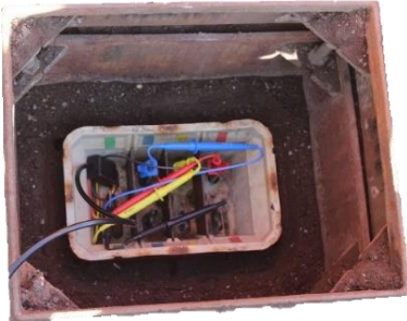
Figure 6.12a: T-P22 connections in the utility link box using clip connectors
