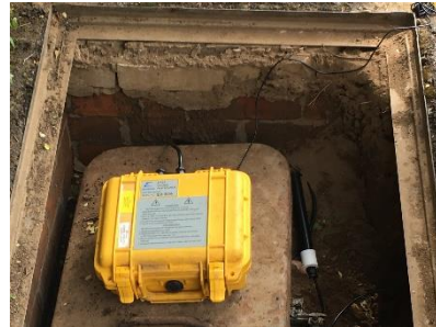
Figure 6.12b: T-P22 laid on top of the link-box bell housing
