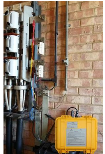
Figure 6.6: T-P22 installed in a substation
