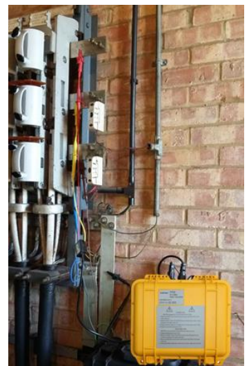
Figure 6.6: T-P22 installed in a substation
